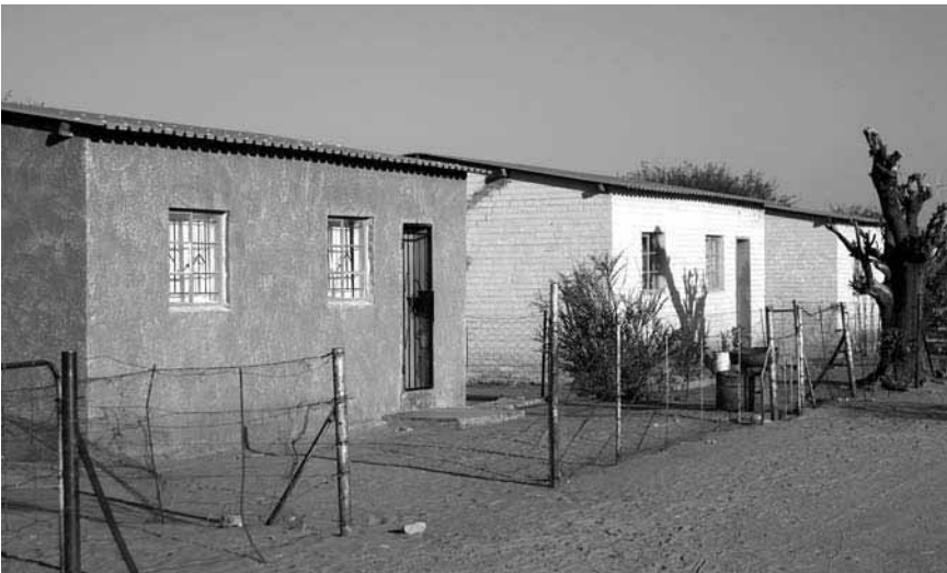
Concrete block houses in the formal area of Epako. Few streets in the community are paved
